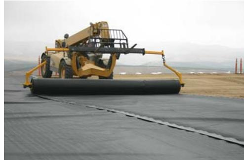
Photos: Liner being installed in mid-September, 2006, at the Santa Maria Regional Landfill. The synthetic liner is about 3/32<sup>nd</sup>s of an inch thick. NHIS will be deposited on top of this layer.
